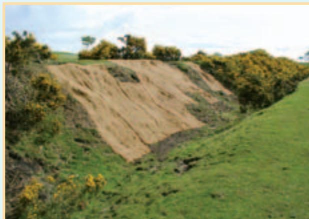
Coir Matting used to stabilise a section of Hadrian's Wall ditch
