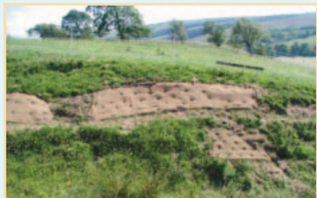
Turf stack repair on completion
