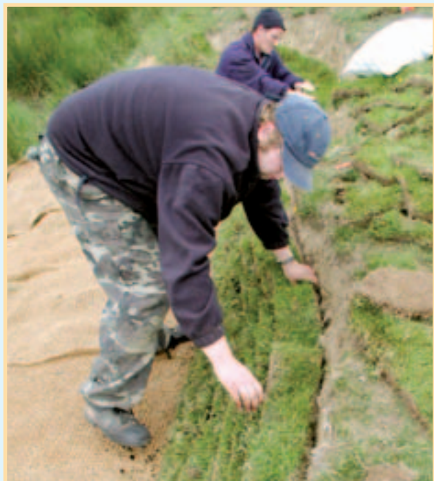
Turf stack repair being constructed.
