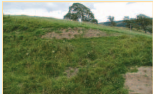
Turf stack repair two months later
