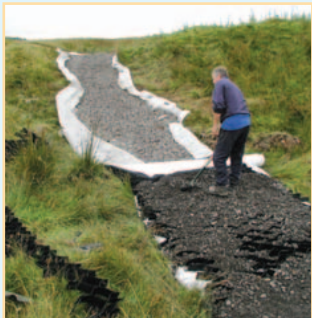
Expandable cellular mesh used to provide vehicle access across Hadrian's Wall Ditch
