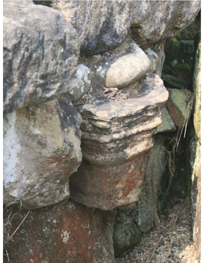
52. A column capital reused in the Willowford bridge abutment
