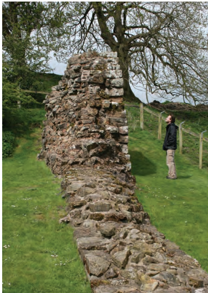
44. Surviving portion of Wall core at Hare Hill
